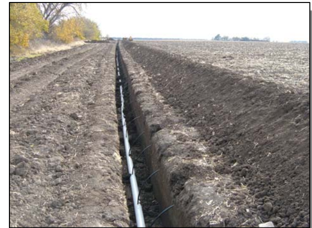
Sub-main feeding one direction
