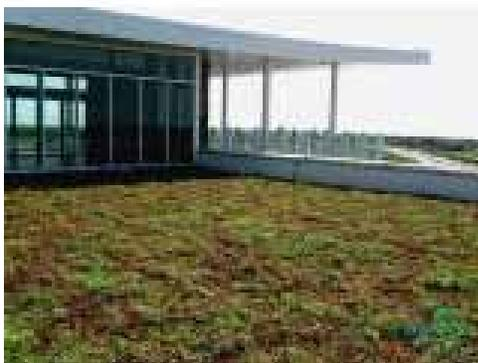
The 'green roof' is an extension of the existing roof which grows light-weight plants and contributes to the buildings lower energy consumption.
