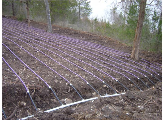
Dripperline is laid in even rows perpendicular to the slope of the field. Note how the tubing passes close to trees that remained in the drip field. Notice the use of flex PVC to transition from the supply and return headers up to the dripperline laterals. This helps to protect the dripperline from damage in poor soils as well as preventing drippers from being placed outside the boundary of the drip field.
