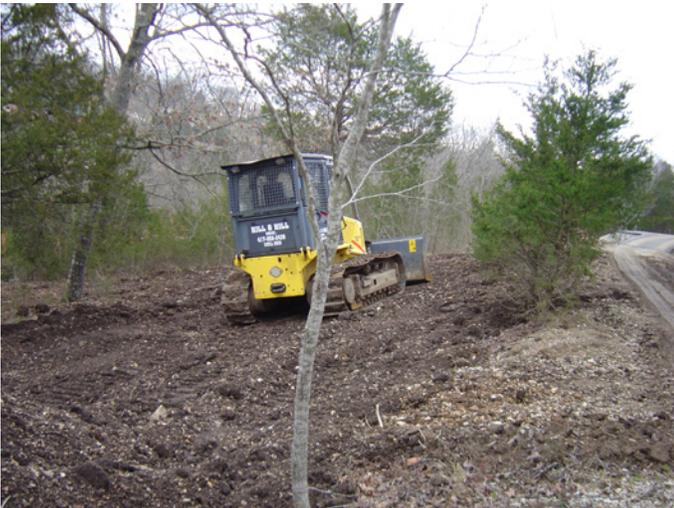
Imported soil is spread across the future drip dispersal field before dripperline is installed. Bringing in soil in 4" to 6" lifts is typical. Total soil depth of approximately 18" was achieved.
